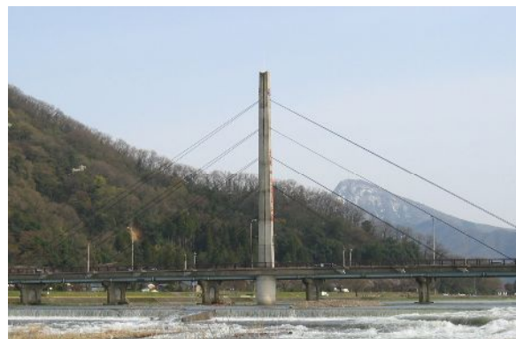
The Bandai Pedestrian Bridge (Echizen City)
