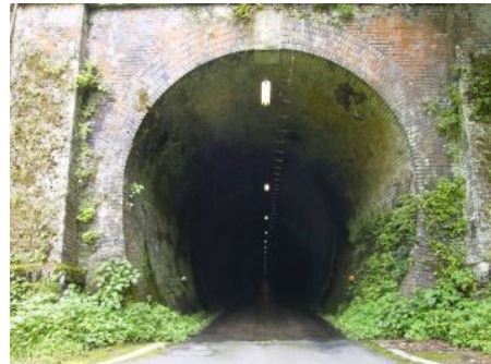
Yamanaka tunnel ①
