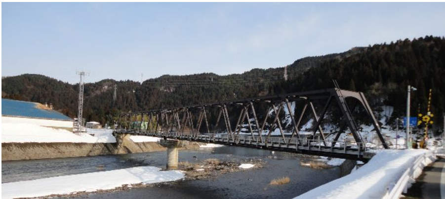
1st Asuwa River Bridge (Abaka-cho, Fukui City)
