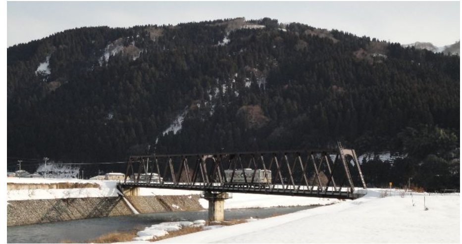
5th Asuwa Bridge (Ichinami-cho, Fukui City)
